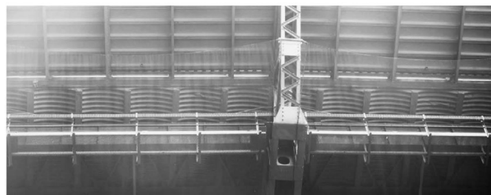
Figure 6. The Sydney Harbour Bridge – Series of 9 arcs supporting the analysed band [1]
