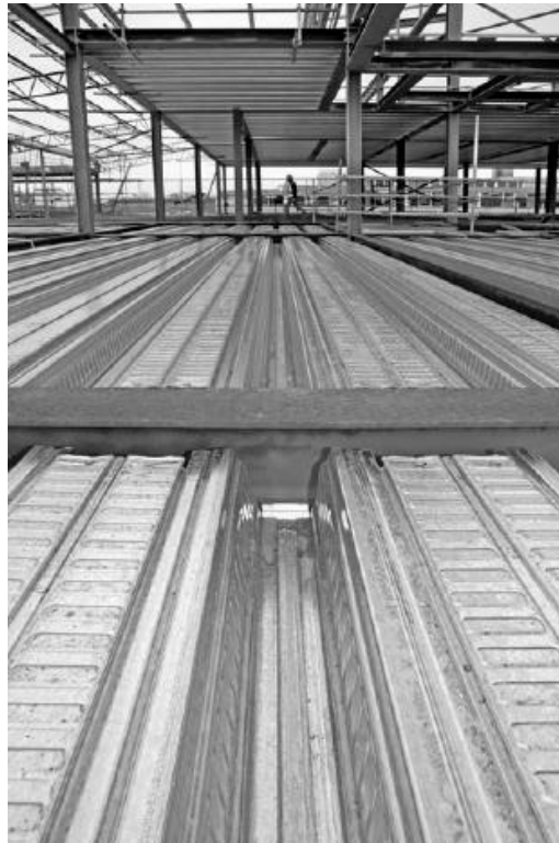
Figure2. The Slimdek composite flooring system.
