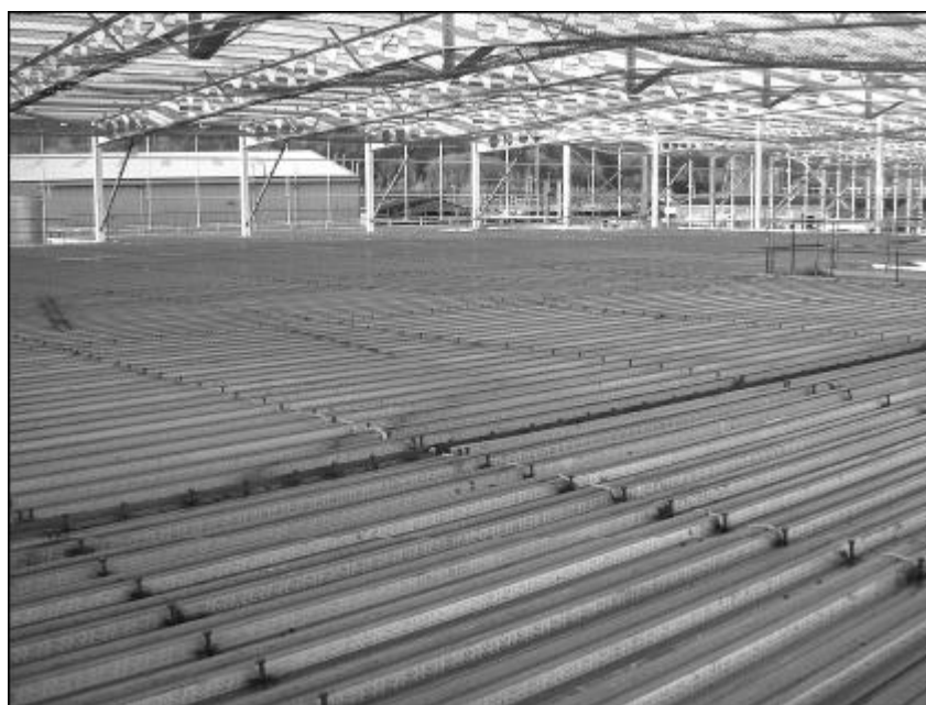
Figure 1. Typical example of a composite floor
