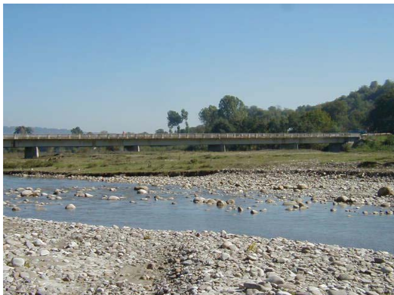
Photo.3 Bridge over Putna river, at Vidra (constructed in 1965)
