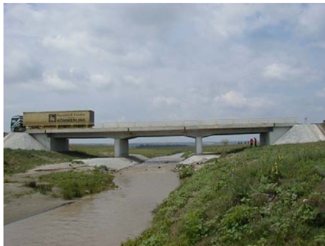
Photo. 1 Bridge over Berheci river, at Berheci (constructed in 1960/rehabilitated in 2002)
