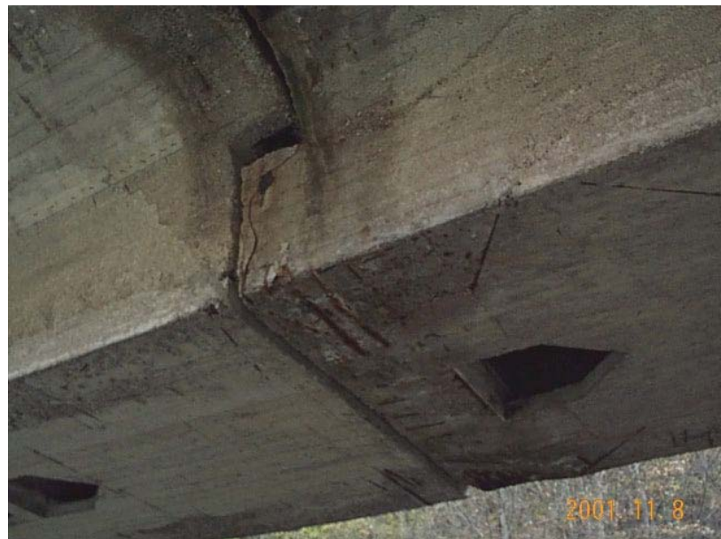
Photo.11 Bridge over Oituz river, at Oituz
