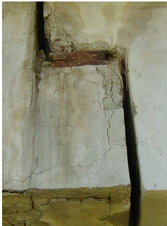
Photo.12 Bridge over Putna river, at Vidra
