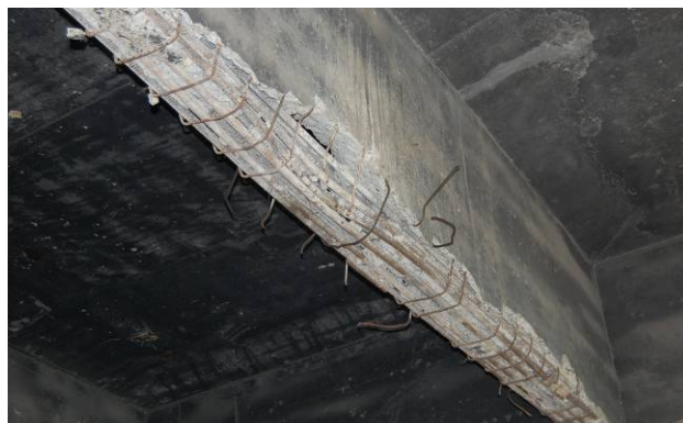
Figure 4. Beam 2 (central beam)
