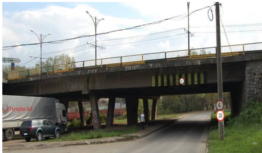
Figure 1. Lateral view towards the first hit beam
