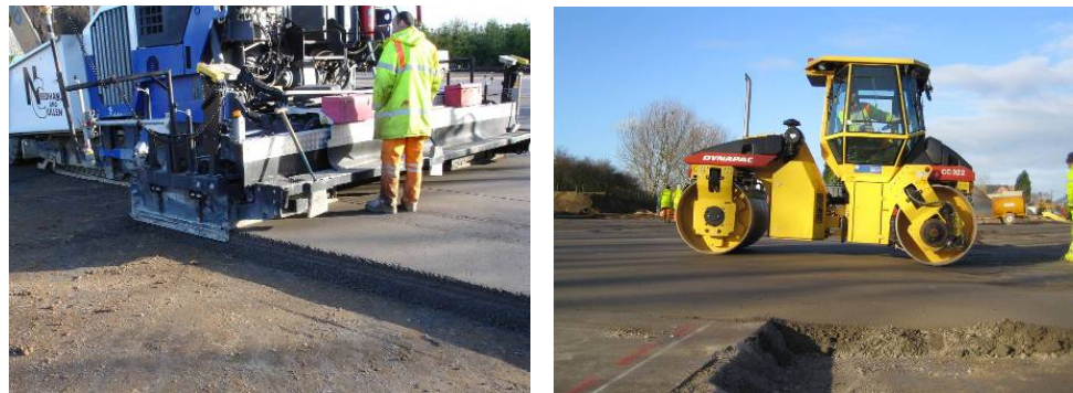
Figure 1: Paving operation and compaction of the pavement by heavy vibratory rollers
