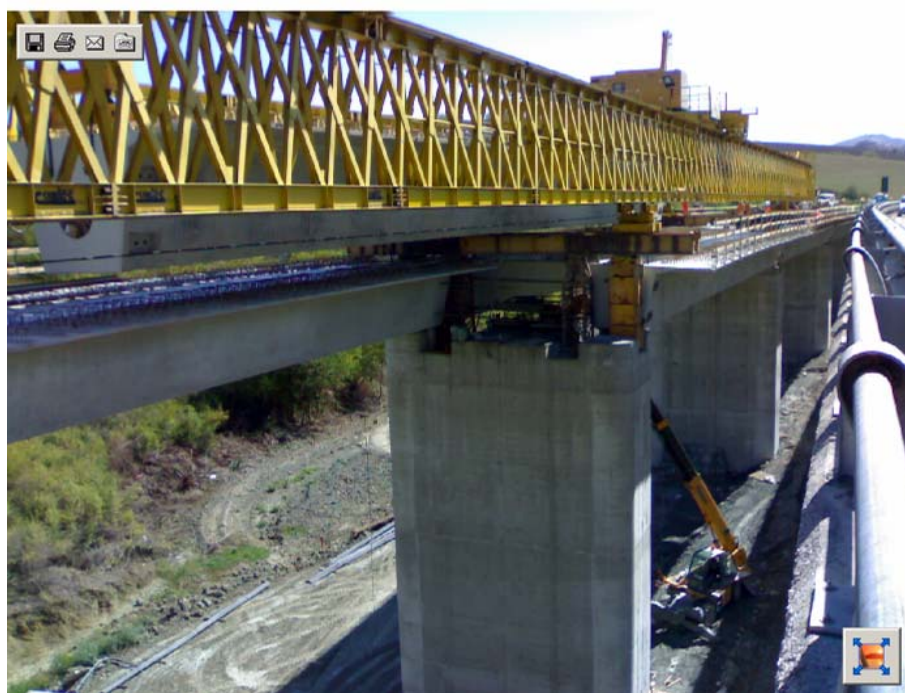
Figure 16. Launching of a beam
