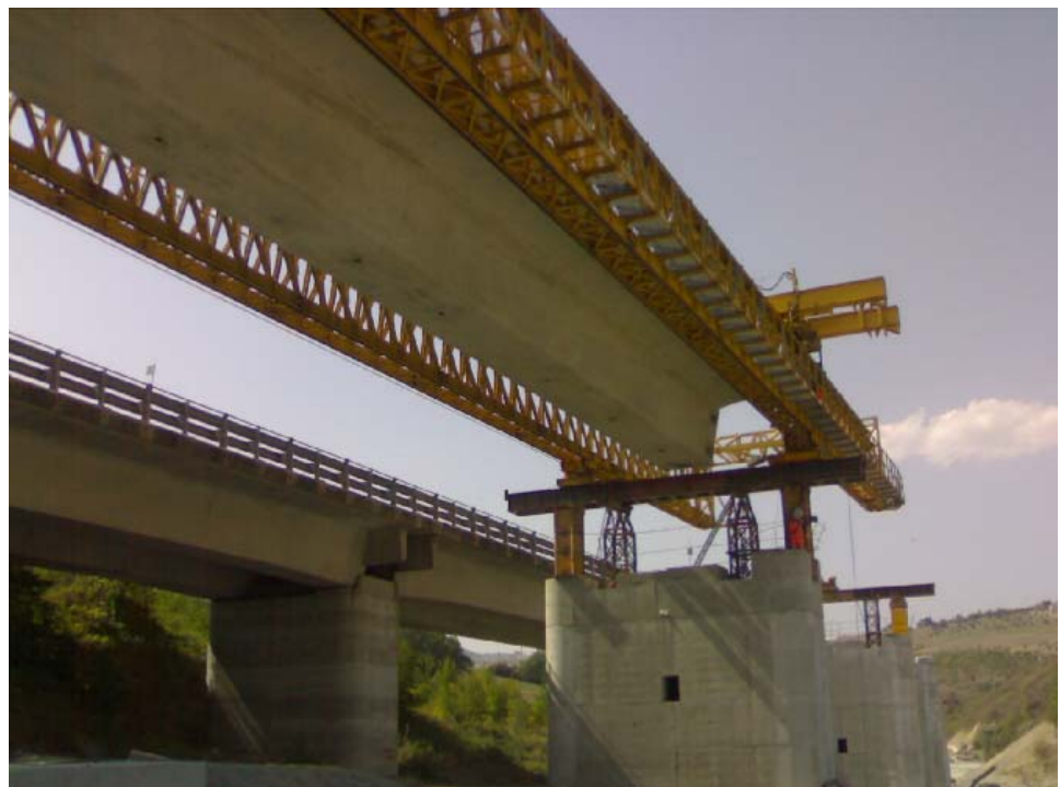
Figure 15. Launching of a beam
