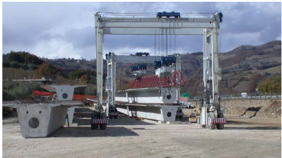
Figure 14. Beams prefabrication site
