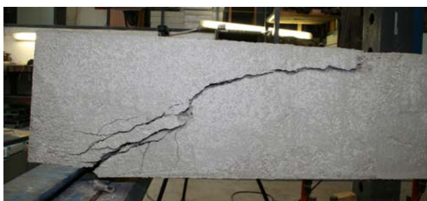
Figure 6. Cracked beam with GFRP shear reinforcement
