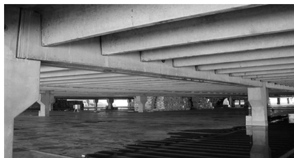
Fig. 2 – Shown Precast concrete beams with installations holes.
