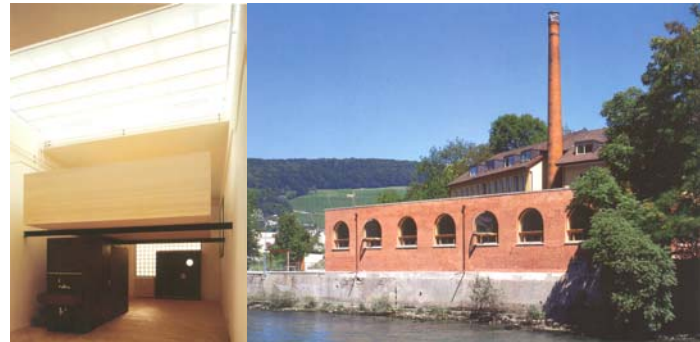
Conversion of water shop into one-room flats – Entebaden, Switzerland
