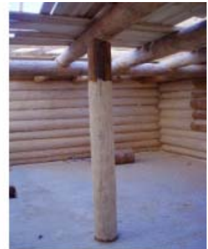
Figure 1. Left –Incorrect construction and insulation of gable; Right –Incorrect placing of vertical element (an adjusting screw is missing)
