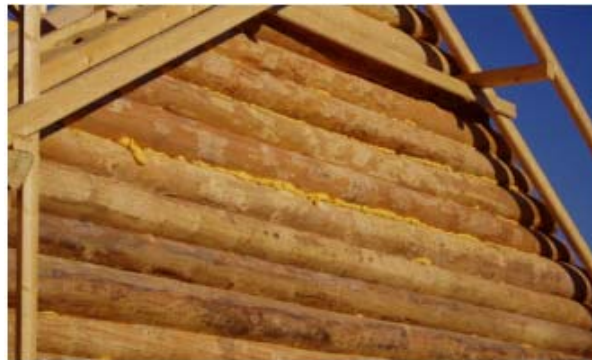
Figure 1. Left –Incorrect construction and insulation of gable; Right –Incorrect placing of vertical element (an adjusting screw is missing)
