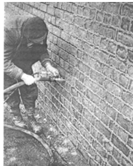
Figure 1. Repointing of the joints
