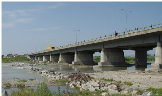
Fig. 3. Elevation of the bridge over Moldova River at Roman, after consolidation
